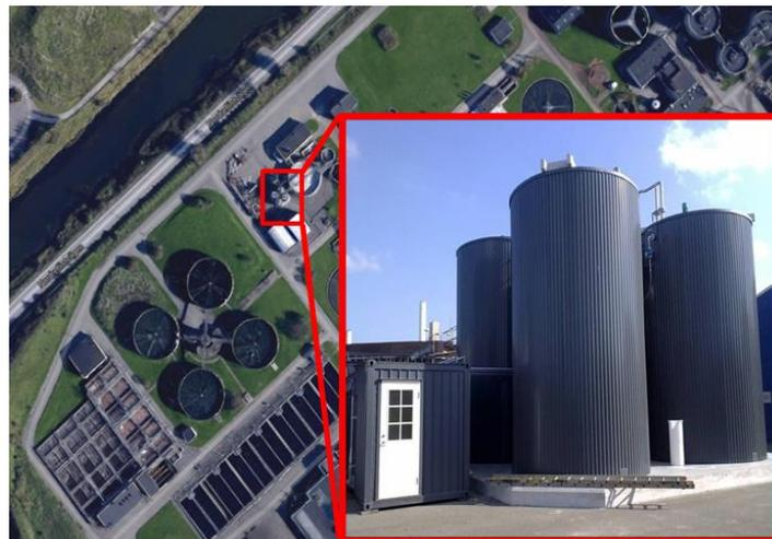
Figure 2: Case Study 2 (WWTP Sjölanda, Sweden), detailed picture of the 2-stage anammox reactor
