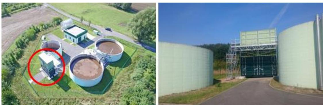
Figure 7: left: Aerial image of the WWTP Westewitz after installation of the filtration plant (encircled in red); right: Front view of the containers of the filtrations plant located between the SBRs.
