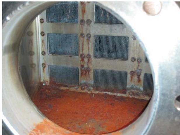
Figure 31: Heat exchange tubes inside the TEG with condensation and rust particles from upstream pipes.
