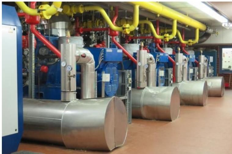
**Figure 4: Four 16-cylinder gas engines (CHP units) installed in the CHP plant in Braunschweig.**
