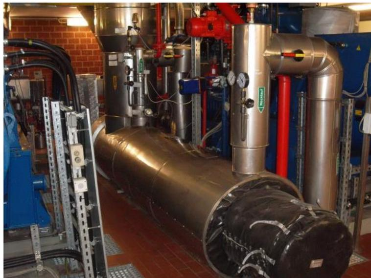
**Figure 7: Exhaust gas heat exchanger of CHP**
